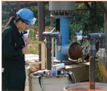
FIGURE 1 | Examples of typical dual carbon canister systems with manifolds to facilitate carbon changeout
