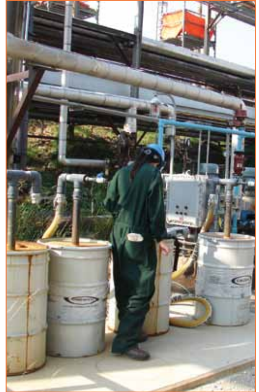
FIGURE 1 | Examples of typical dual carbon canister systems with manifolds to facilitate carbon changeout
